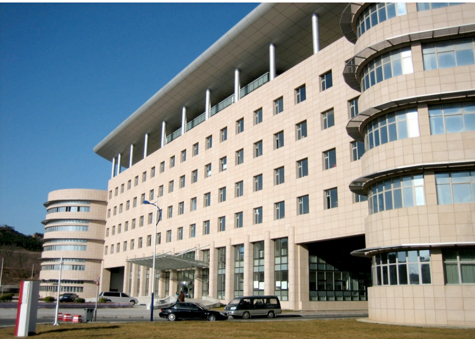
Constructed Gateway building
