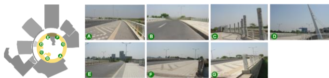
Figure 10. Bridges Over Huanhu Road
