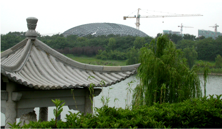
The Science Centre under construction
