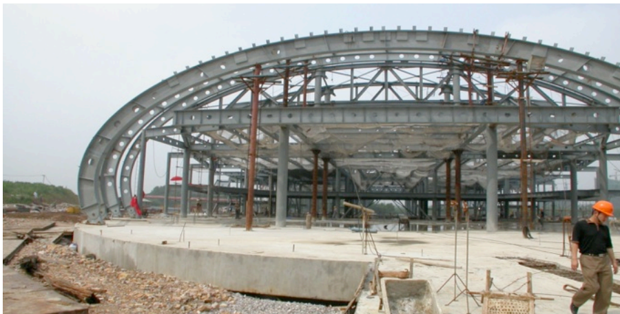
The structural system
