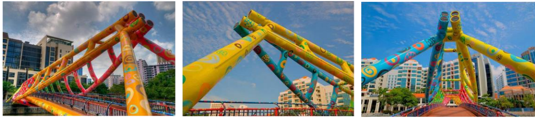
Figure 15. Alkaff Bridge (Singapore's Art Bridge), Singapore Designed by Filipino artist Pacita Abad
