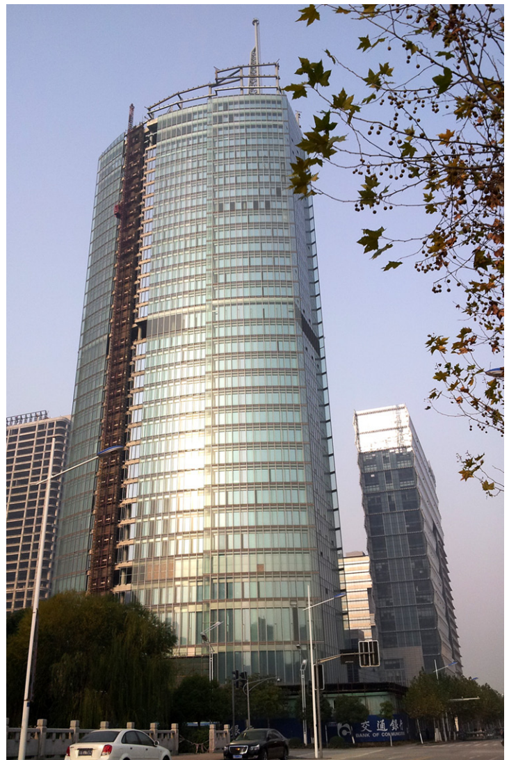
Building under construction
