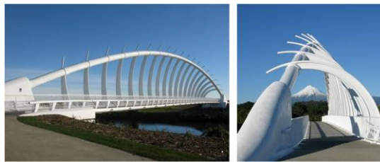
Figure 19. Rewa Rewa Bridge, New Plymouth, New Zealand
